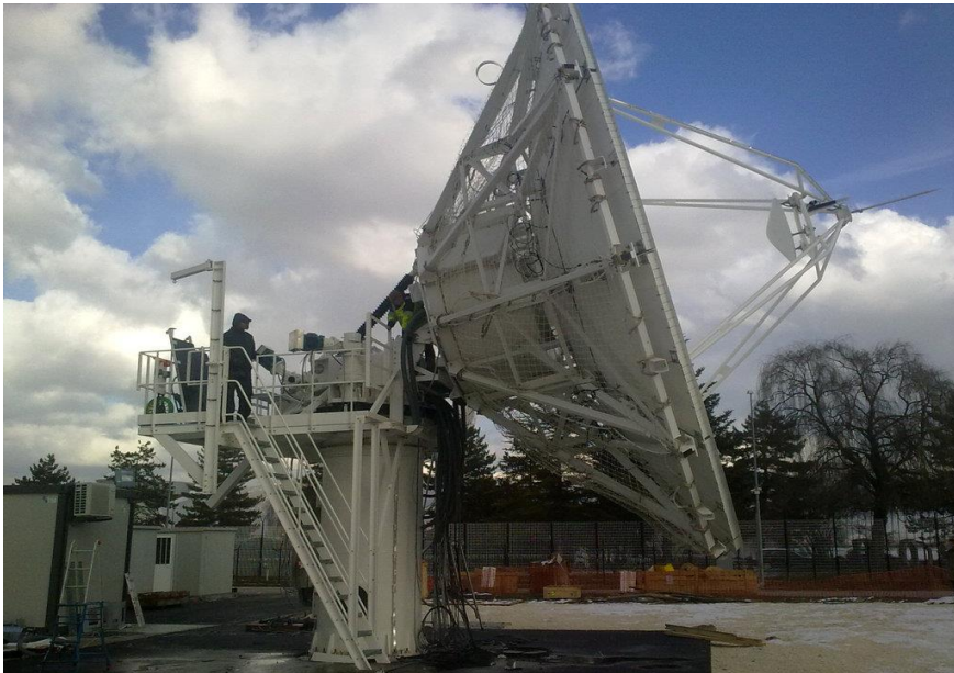
9 mt Ka Antenna of IT civilian Gateway located at Fucino Space Center
